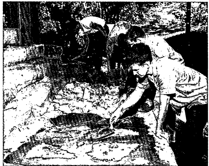
Students Constructing Pathway
